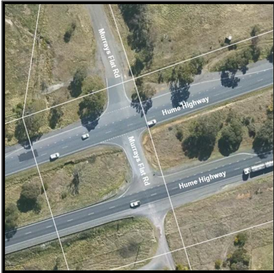
Photo 4: Aerial photo of the 2-staged intersection with Hume Highway and Murrays Flat Road
