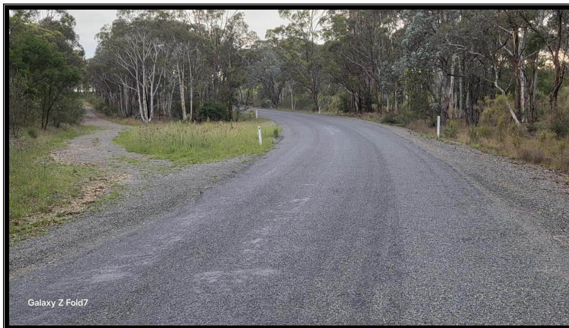
Photo 7: Carrick Road – facing east
