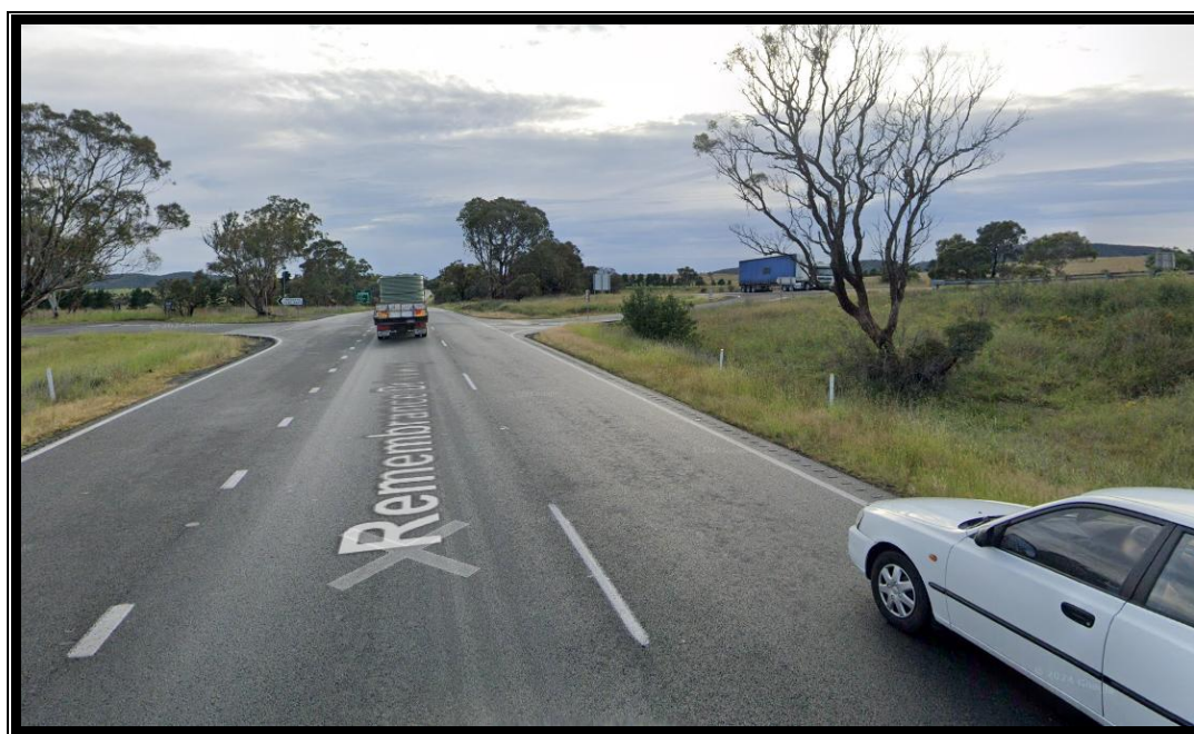
Photo 3: Hume Highway at its intersection with Murrays Flat Road – facing east
